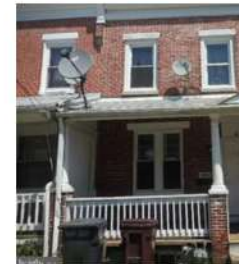
1928 S CAMAC ST.
